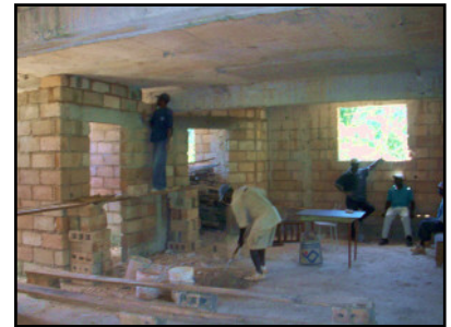
Office walls being finished
